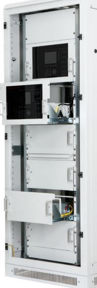
power supply module fail, two additional modules ensure continued operation of the fire alarm control panel.
